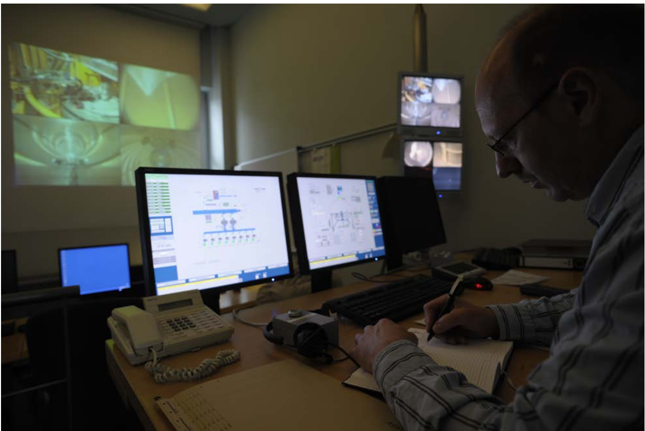
Figure 2.7: Control room of the Bremen Drop Tower.
